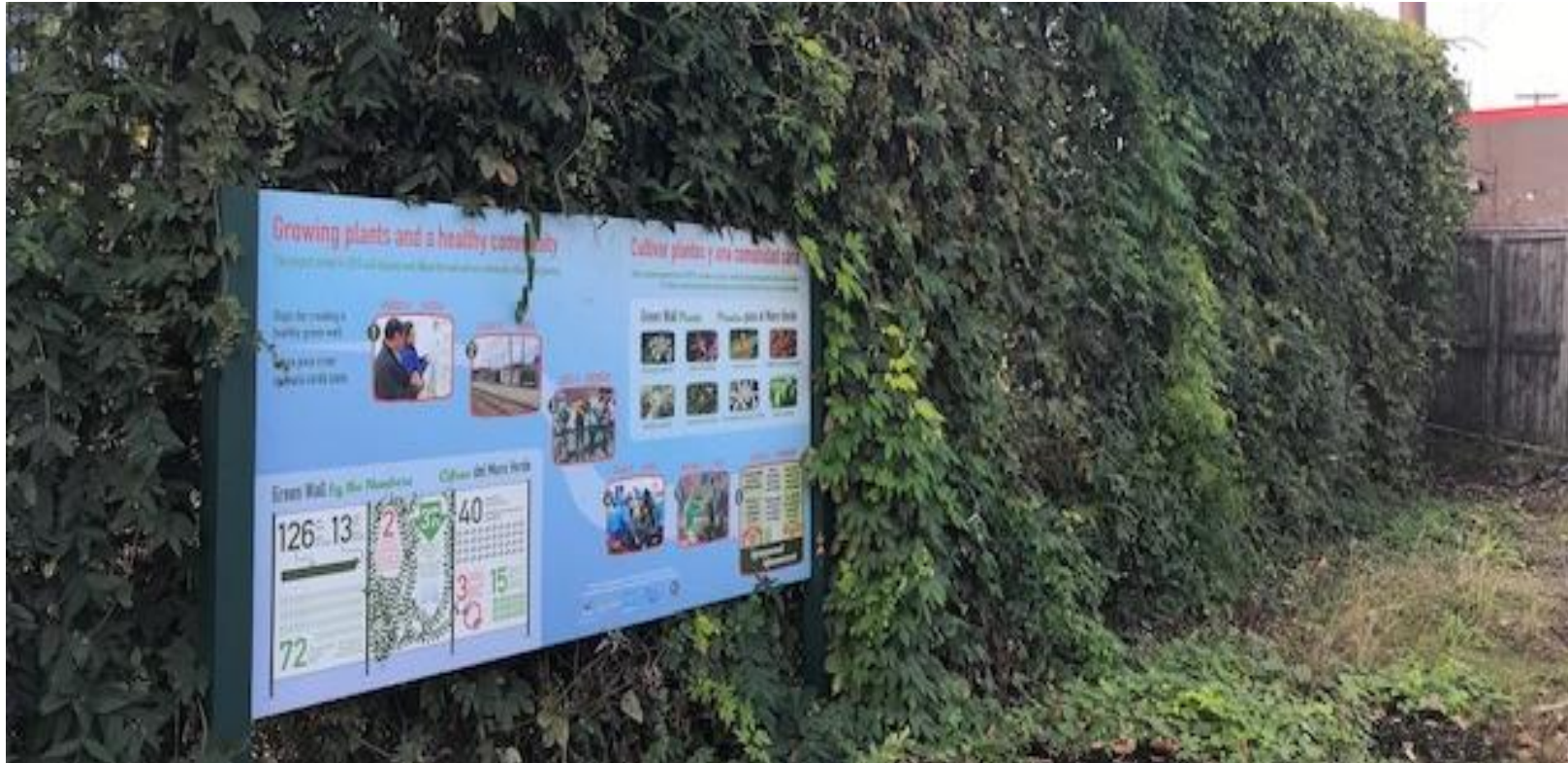
FIGURE 14: A GREEN WALL IN SEATTLE'S GEORGETOWN NEIGHBORHOOD, HELPING TO CAPTURE POLLUTANTS AND RESTORE LOCAL HYDROLOGY (PHOTO CREDIT: DUWAMISH ALIVE)
