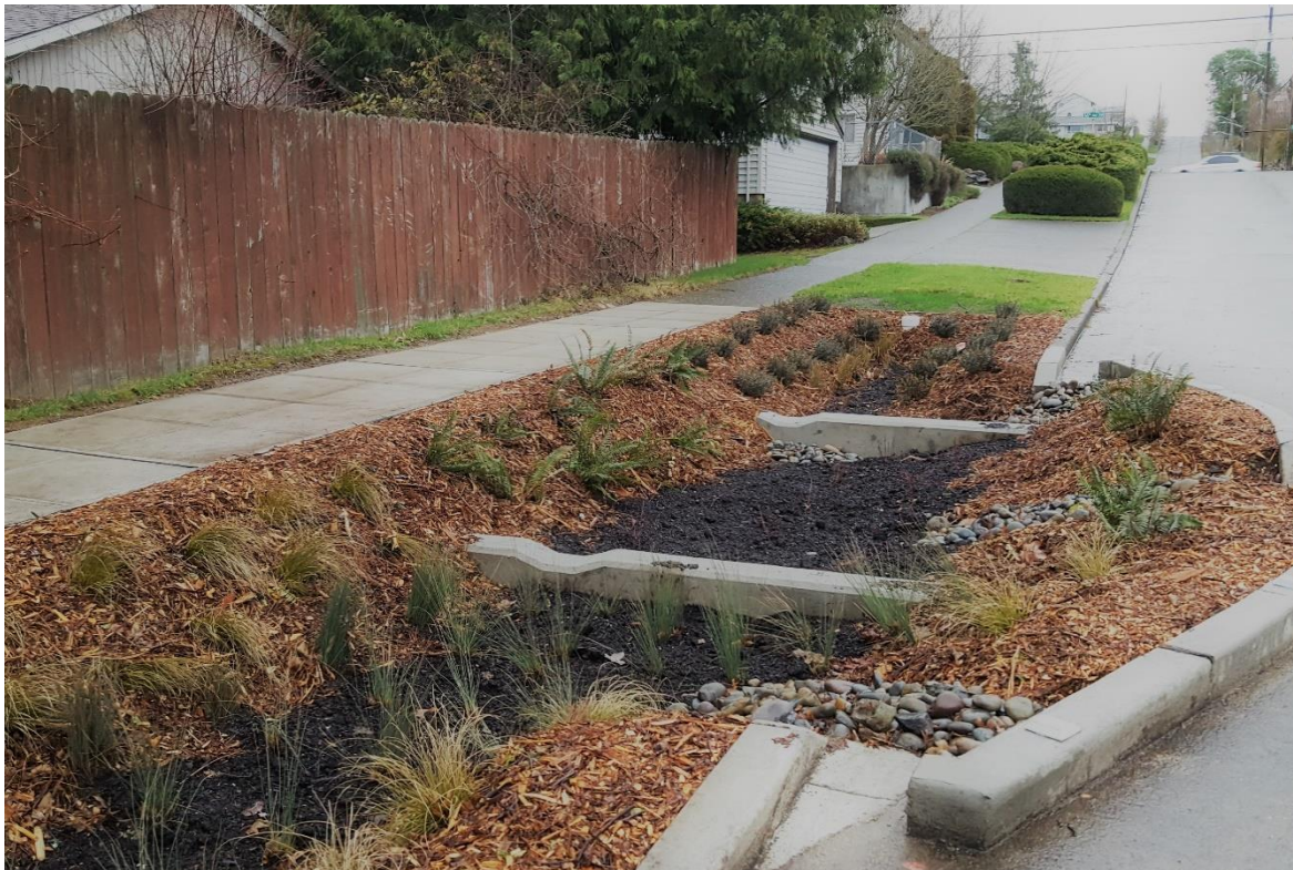
FIGURE 13: GREEN STORMWATER INFRASTRUCTURE IN THE DELRIDGE NEIGHBORHOOD (PHOTO CREDIT: CITY OF SEATTLE)
