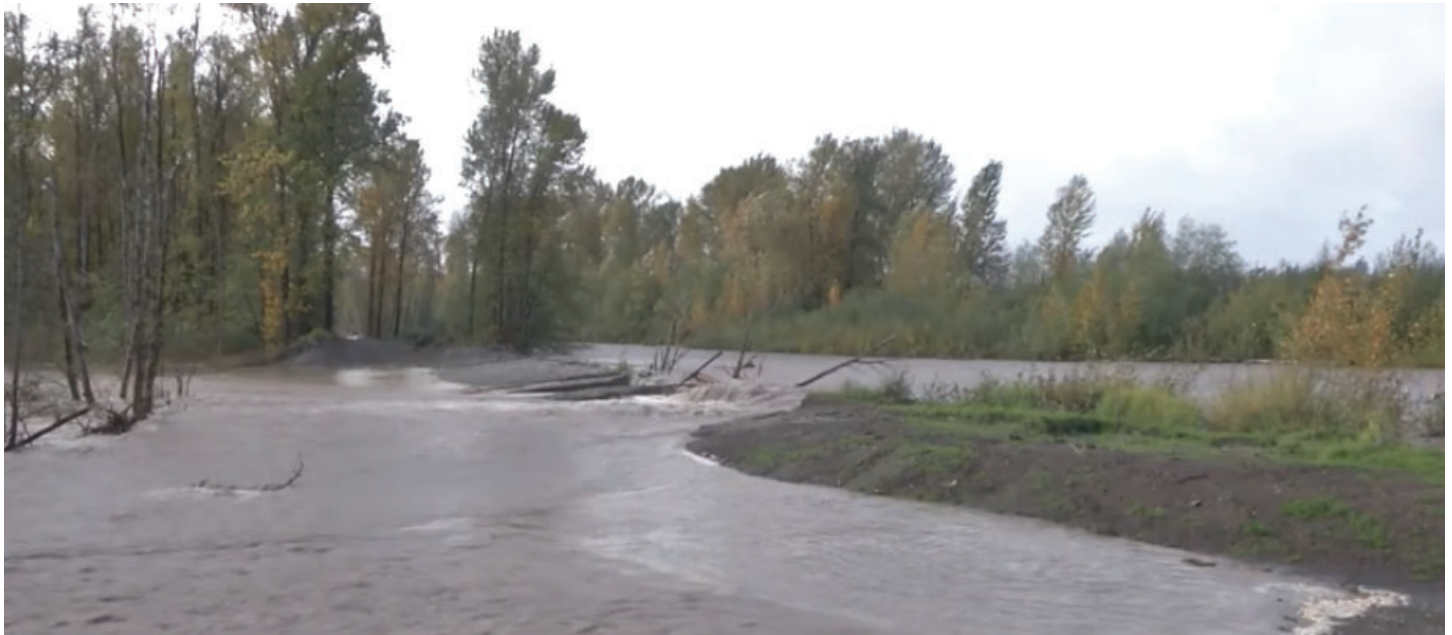
Figure 12. October 2017 Inundation in Countyline Levee Setback Project Area
